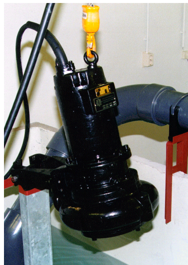
Figure 4: Landustrie DECR 20-8 submersible pump
